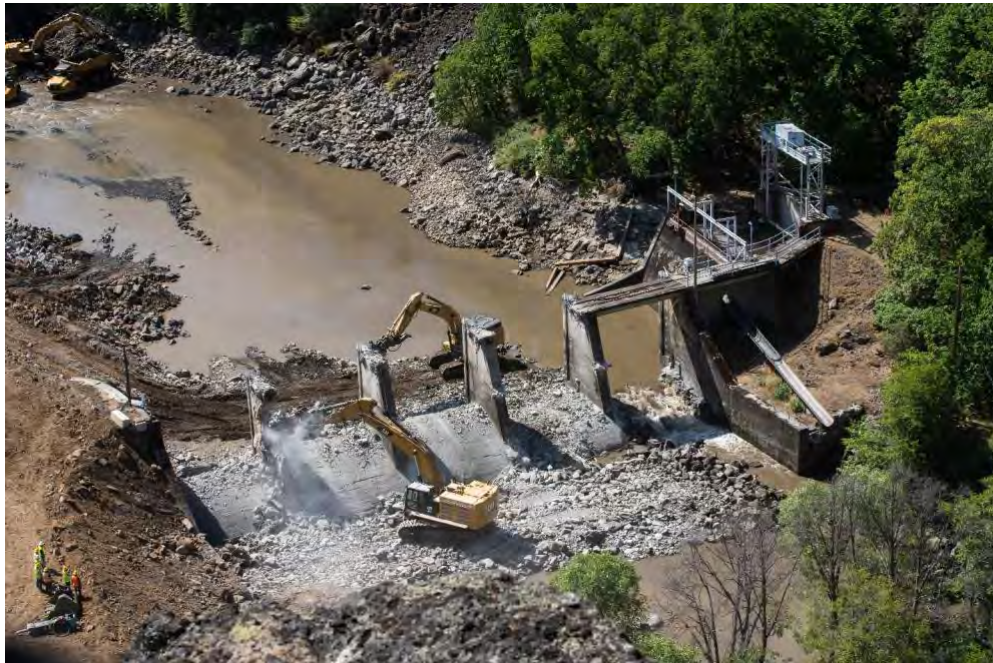
Decommissioning and removal of Copco 2 Dam (Credit: Shane Anderson)
